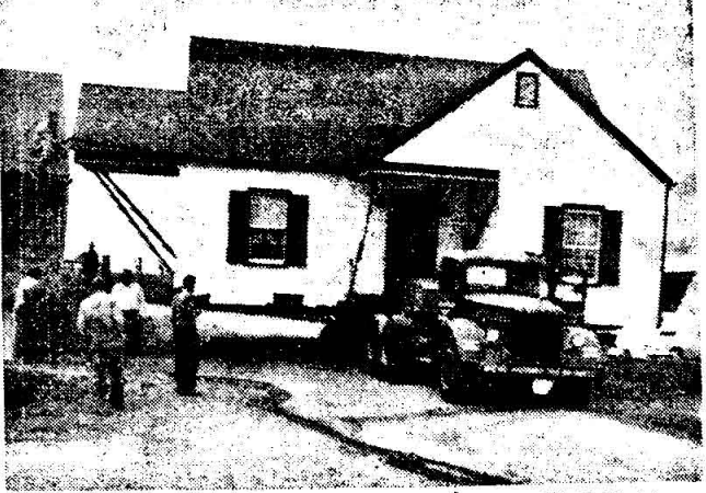
(Staff Photo) MOVE OVER BUD — The house of A. H. McMahan, about two miles west of Marion on Rt. 11, was moved Friday by Joe Guyton for the construction of the dual lane highway to come into Marion. The house had to be moved about one quarter of a mile to a new position. The big pain for Joe was to move the house past another house on the way and miss going over a bank.
