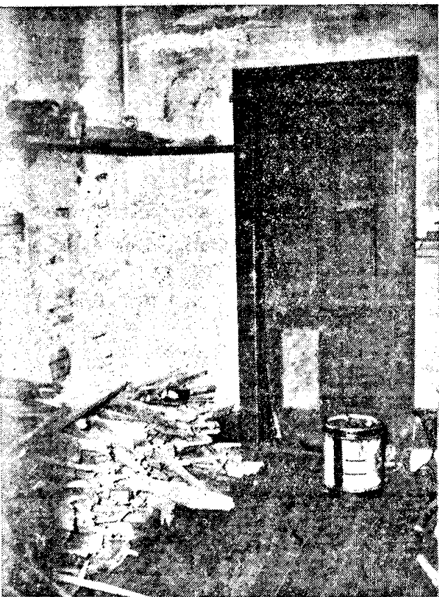
STORAGE ROOM — This is the storage room. The small boys who cut the wood for the stoves use this room to store it until used. In this room notice the plaster that has broken off the walls and the door. The door has been split at the bottom and there is no lock on this room.
